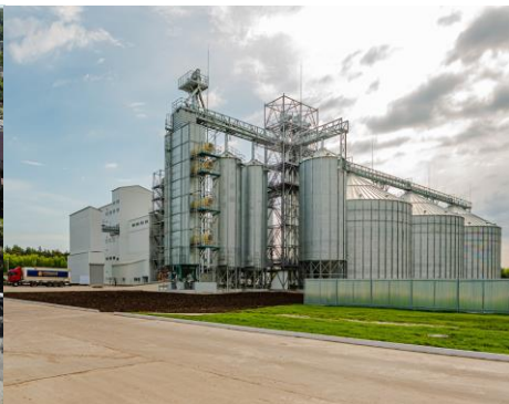
Sakhalin Feed Mill
