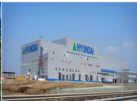
Plant of electrical equipment «HYUNDAI» in Artem
